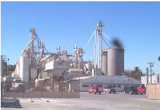
Grain Silo Complex on Second Avenue
