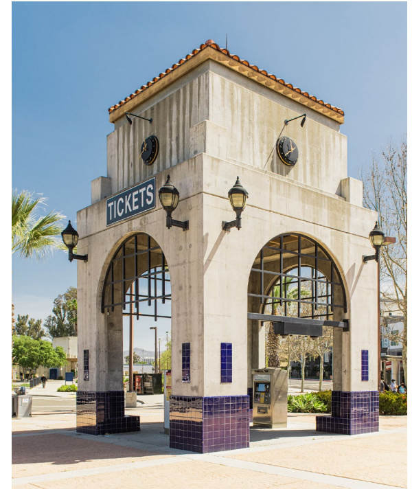
Transit Center. Source: City of Escondido, 2021
