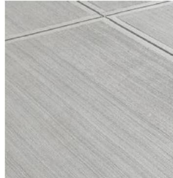
Concrete Flatwork broom finish
