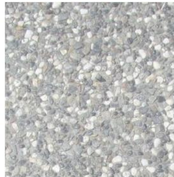
Concrete Flatwork heavy aggregate finish
