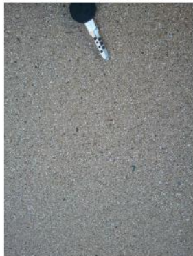
Sand Finish Concrete - #5 TopCast with Davis 'Sandstone' color
