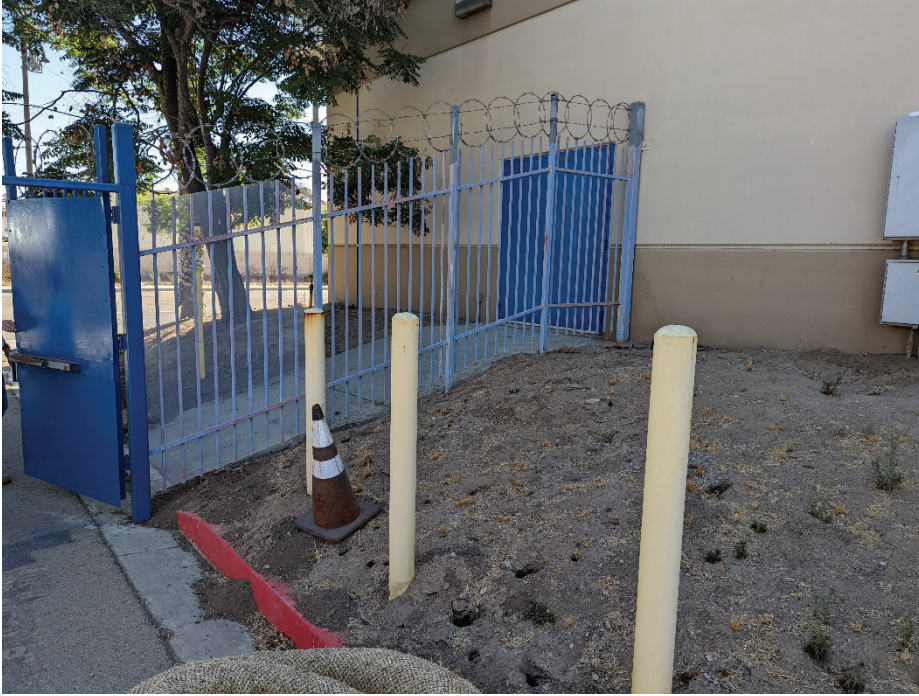
Photo 5: Existing conditions within Project site along the northern boundary. View northeast.
