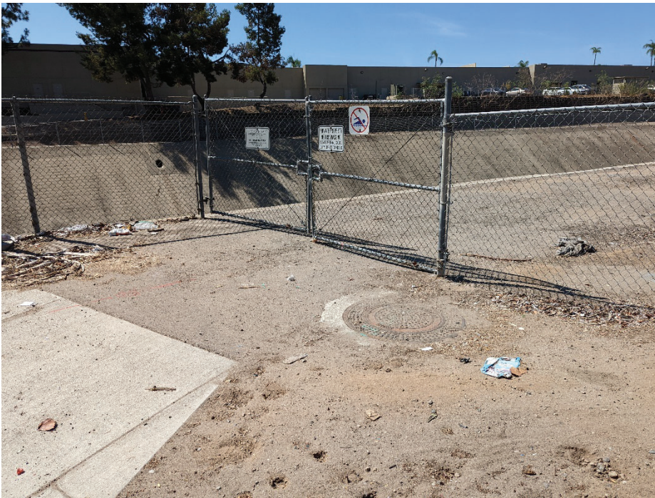
Photo 8: Existing conditions immediately outside Project site near eastern parcel corner. View south.
