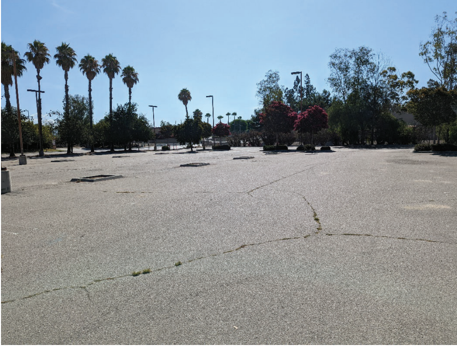
Photo 3: Existing conditions within Project site. View east-southeast.
