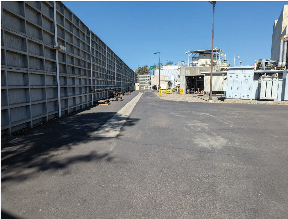
Photo 4: Existing conditions within Project site along the southern boundary. View west.
