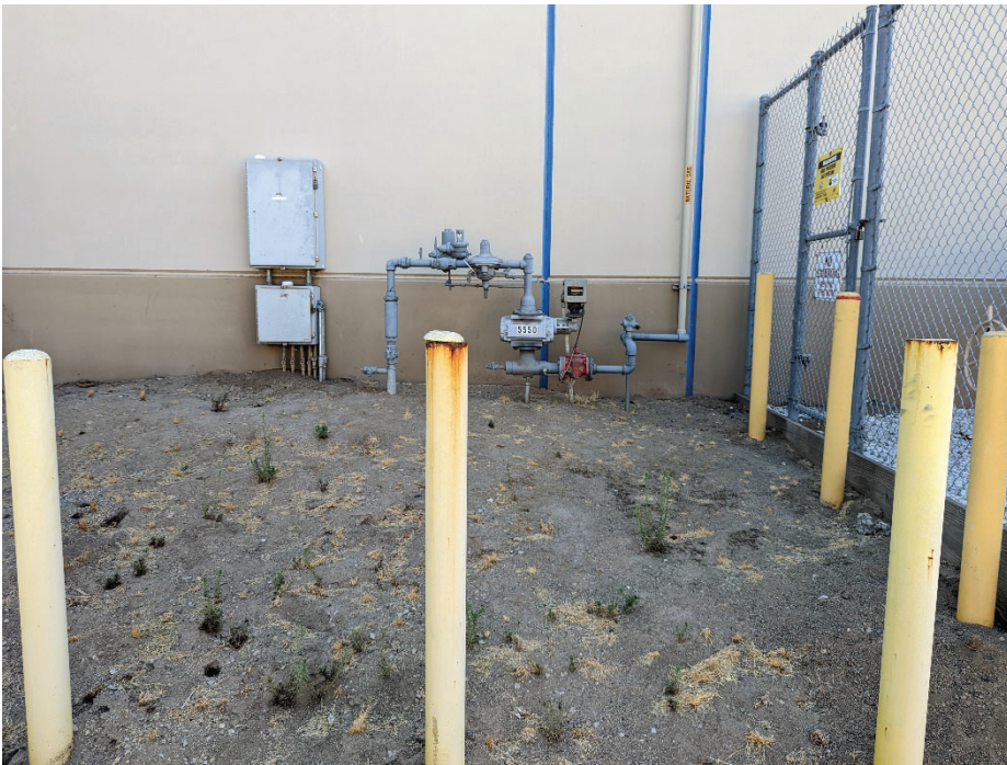
Photo 6: Existing conditions within Project site along the northern boundary. View southeast.
