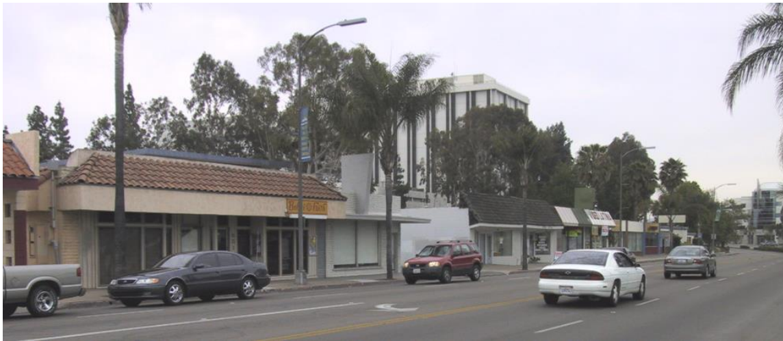
Palomar Hospital anchors the west end of the parkway adjacent to downtown Escondido
