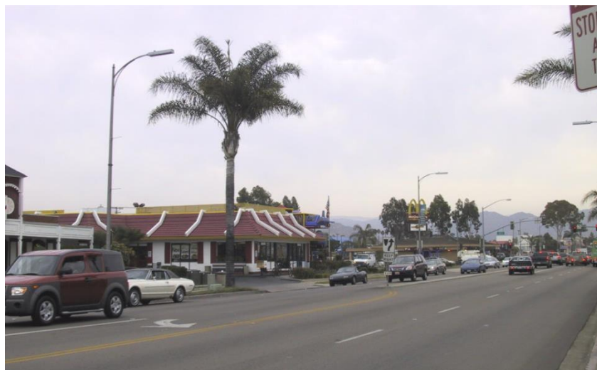
Mid-block left turn lanes, which facilitate access to individual businesses, may impede traffic flow
