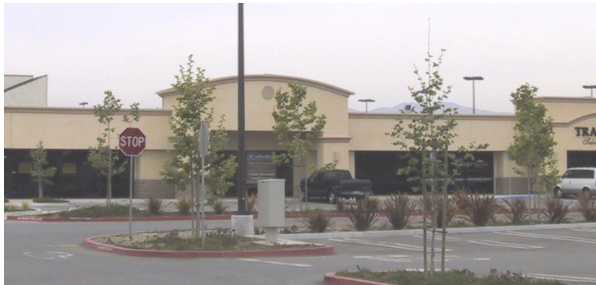
This comprehensively designed center incorporates large cornices, arched rooflines, covered arcades and simple building lines
