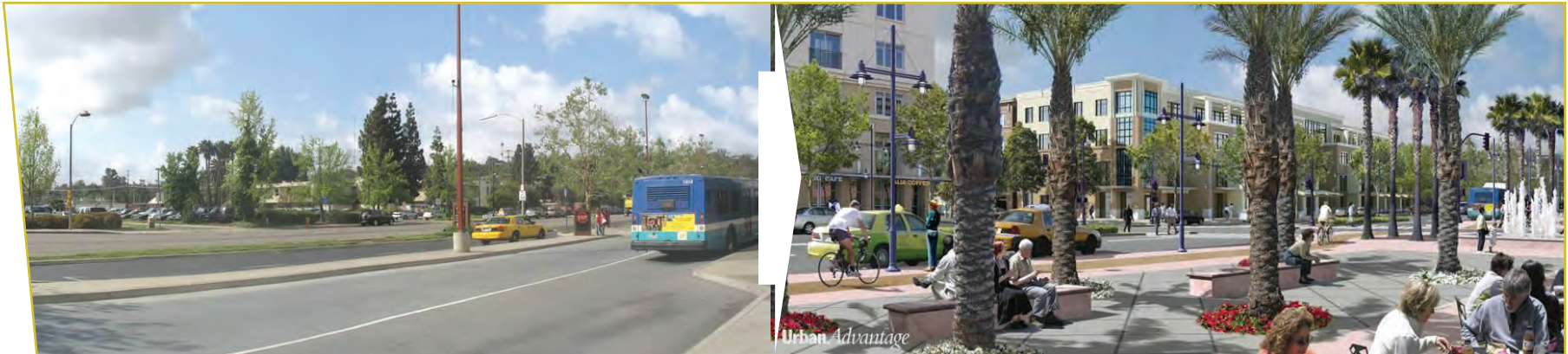
A “before” and “after” example illustrating how smart growth mixed use transit oriented development can transform the area around Escondido’s multi-modal transit station into a dynamic employment center. (General Plan page 15)
