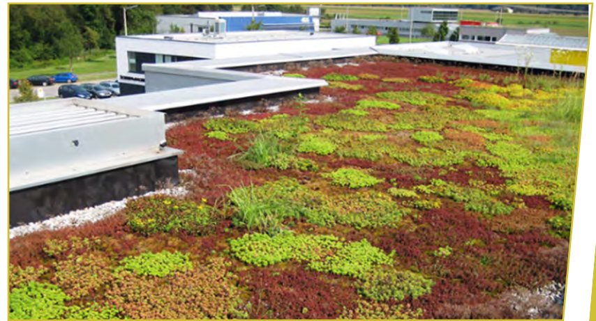
Extensive example on a commercial building
